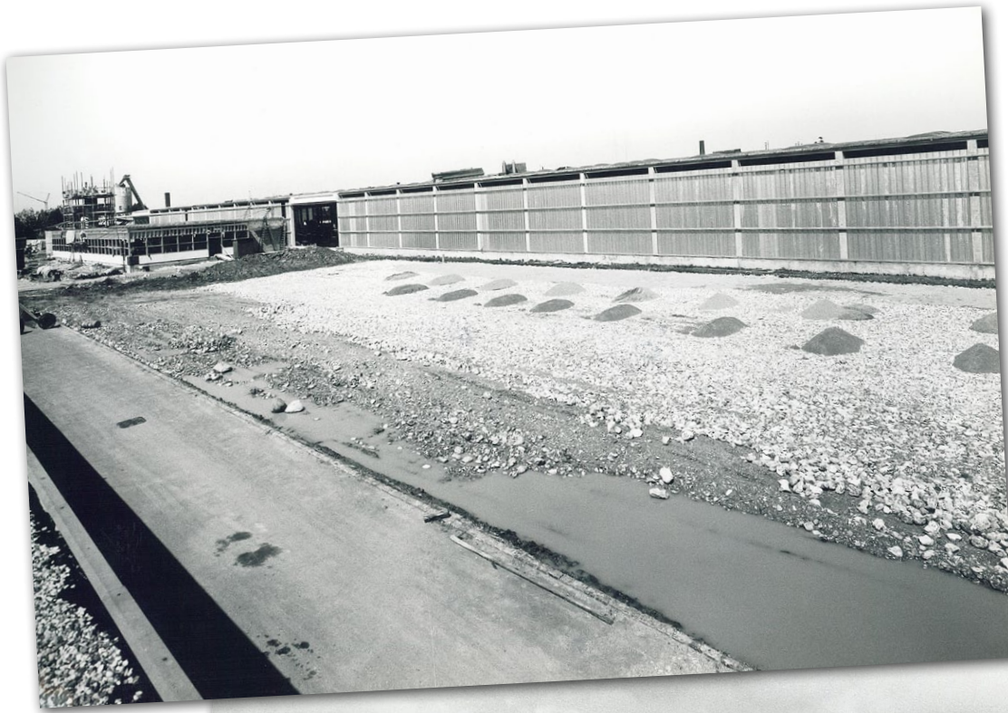
Construction of the central warehouse at Rørvang, June 1965.
